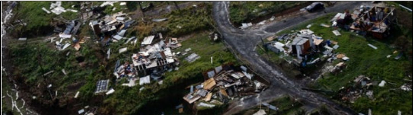
Damage in Puerto Rico after Hurricane Maria. Photo: CNN Money
